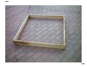
After the boards are nailed together (like it is shown above) paint the outside using white latex paint. This provides protection for the wood from water, light, bacterial and fungal damage. Now line the frame with the plastic, nailing it on the borders using small nails.
